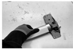
Test the Exit Device to make sure proper contact of RX7700 switch trigger.
